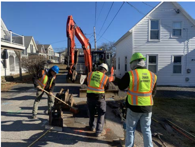
Crew excavating test pits on High Street.
