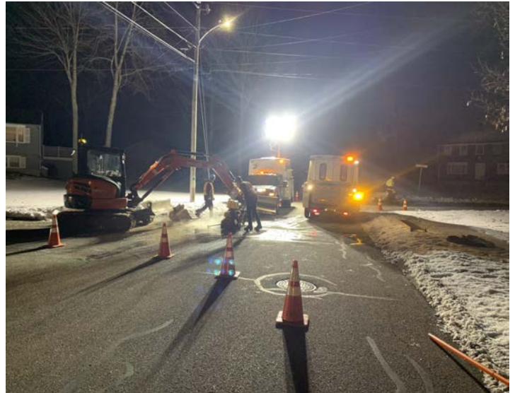
A job zone for an emergency valve repair.
