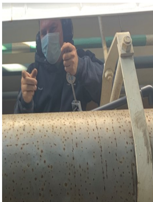
A staff member replacing overhead piping.
