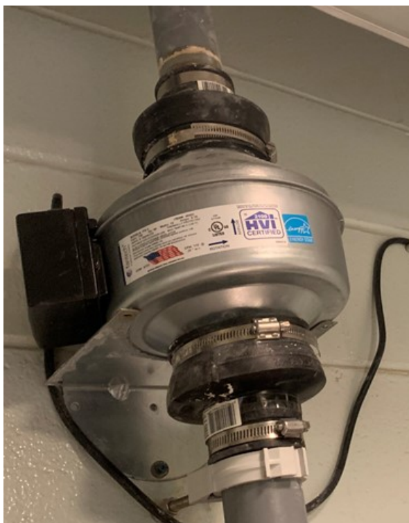
A new ventilation fan was installed at the treatment plant.
